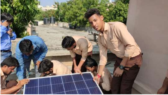
Solar Technician on OJT-Installing Solar Panel.
