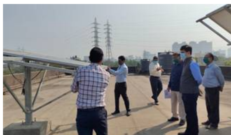
Solar Panel installation – NSTI Mumbai
